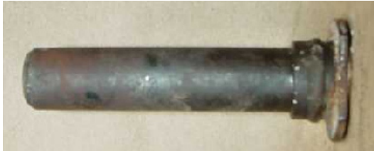
Figure 34. Leading Pin with Light Corrosion
